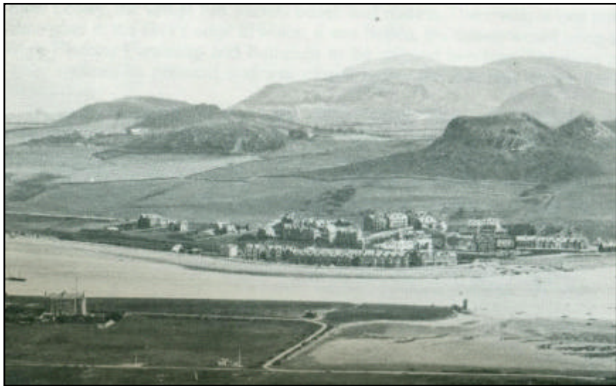
Figure 5. View of Deganwy, Marine Crescent, Deganwy Castle Hotel, Terraces along Station Road with large houses along Glan-y-Mor Road & the start of York Road with lots of open fields behind
