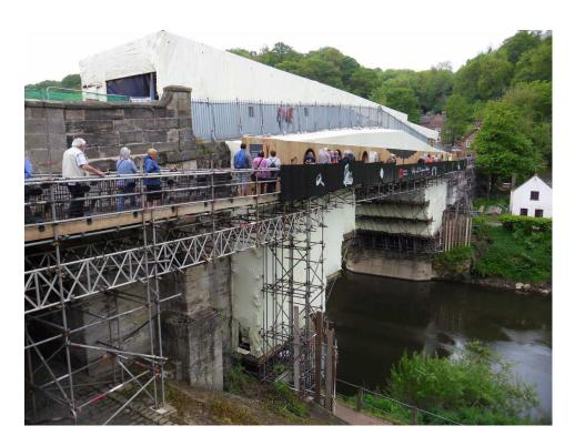
However, although the bridge itself was enclosed with scaffolding and sheeting, a walkway had been created alongside the bridge to enable visitors to view the work taking place which would not usually be visible. English Heritage guides were readily available to explain the repairs and point out the intricate ironwork and missing or damaged sections of the arch.
