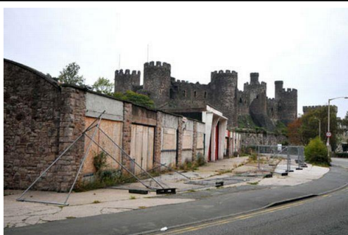
Billington's garage before demolition in 2012
